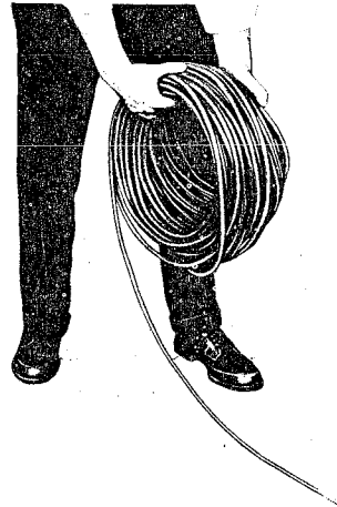
Fig. 3 — Paying Out Cable
